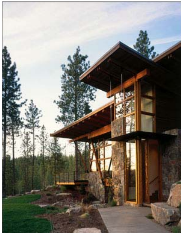
Piers made of local basalt stone support the structure and follow the contours of the land.
